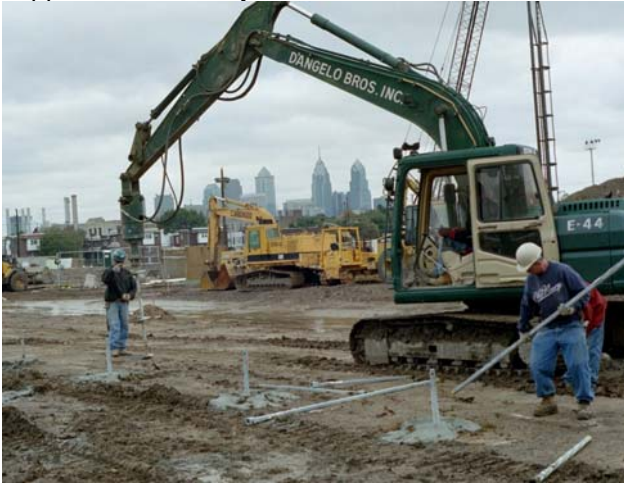
Figure 10 Phase II & III Excavator and Torque Motor
