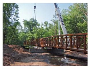
After the bridge sections were connected, the bridge was then lifted and placed into the final position on the concrete abutments. Installation of the bridge from when it was brought to the site to when it was completely installed took less than 4 hours.
