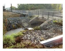
Stone riprap was placed at both abutments and along the channel. A gabion wall [wire mesh encased riprap] was installed along the fence line to act as a retaining wall.
