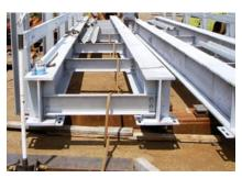
The bridge superstructure was constructed of steel stringers with diaphragms equally spaced along the length of the bridge. The bridge was prefabricated in two 8 foot wide sections, each measuring 39 feet long.
