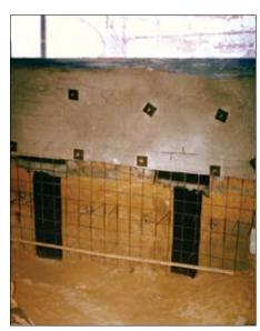
restricted footprint was accessible with extendable sections of the Soil Screw® Retention Wall System. As little as 1 foot of freeboarding space was available in some zones.
