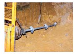
termination. A 4 x 5 ft. grid was determined for use on this  $100 \times 50 \times 21$  ft. excavation. Boring logs showed the screw anchors were installed in firm and very firm, silty coarse-to-fine sand with Standard Penetration Test results typically from 10 to 20 blows per foot. Preloads of 20,000 lb. tension were selected for one to two tests per site.
