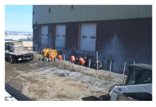
load to supporting soils below the existing basement wall foundations. A total of 35 AB Chance Pulldown Micropiles were installed to a minimum depth of 25-ft in conjunction with Geopier Intermediate Foundations to provide foundation and floor slab support adjacent to the existing warehouse basement.
