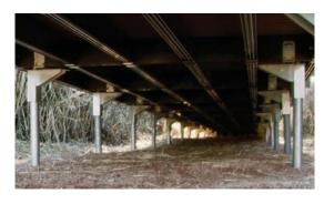
ALL ALUMINUM structural framing and railing members. 1000PPSF rating. For consistently strong and positive connections at critical points in the framing with no possibility for poor workmanship.
